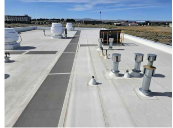
UPPER ROOF AREA WALKWAY & VENTS LOOKING SOUTH
