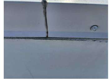
EXIST. METAL FLASHING UPPER ROOF AREA
