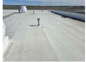
UPPER ROOF AREA WALKWAY & VENTS LOOKING NORTH
