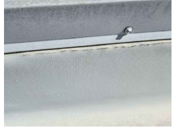
EXIST. METAL FLASHING UPPER ROOF AREA
