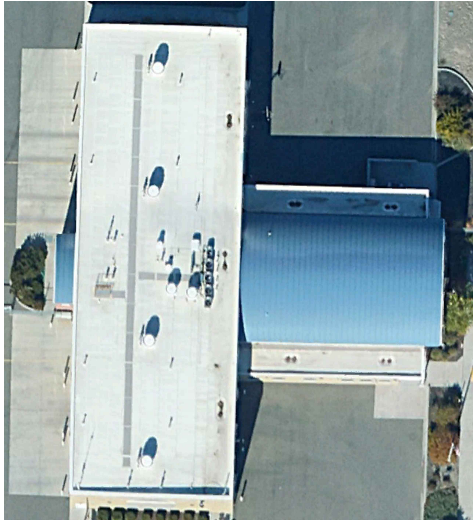
AERIAL VIEW OF UPPER AND LOWER ROOF AREAS
