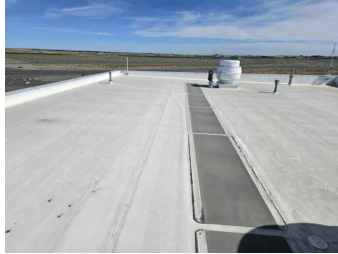
UPPER ROOF AREA WALKWAY & VENTS LOOKING NORTH
