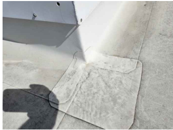
EXIST. TPO FLASHING UPPER ROOF AREA
