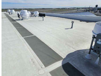
UPPER ROOF AREA WALKWAY & VENTS LOOKING NORTHEAST
